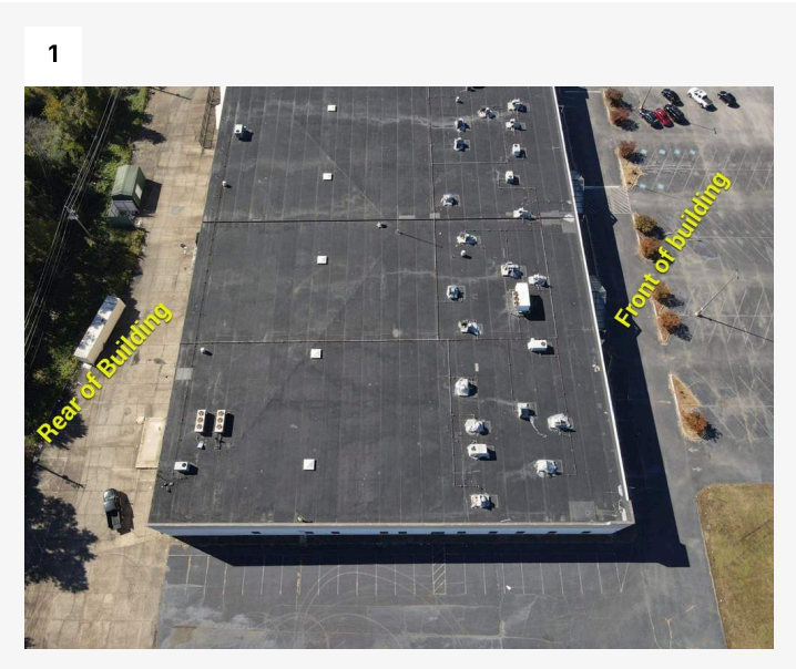
Image 1 Northeast end of the building, visual reference image. Building front is to the right, rear to the left.
