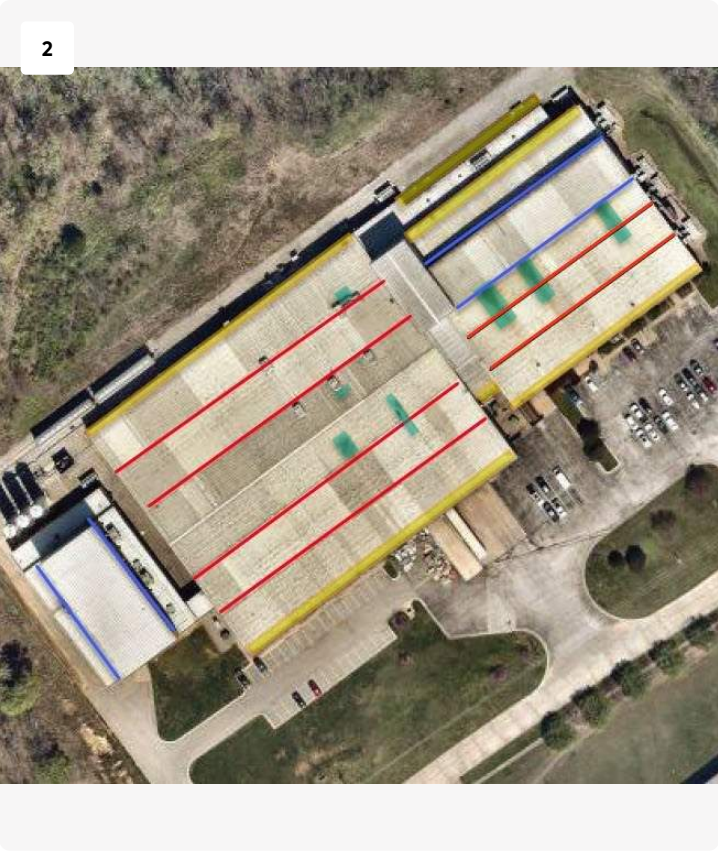
Overview of building
